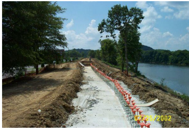
Figure 4-6. Metro Center Levee Rehabilitation
