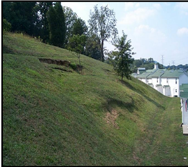
Figure 4-10. Evidence of Landslides
