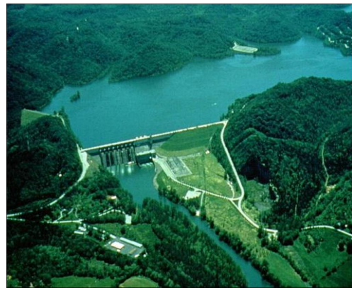
Figure 4-4c. Center Hill Dam
