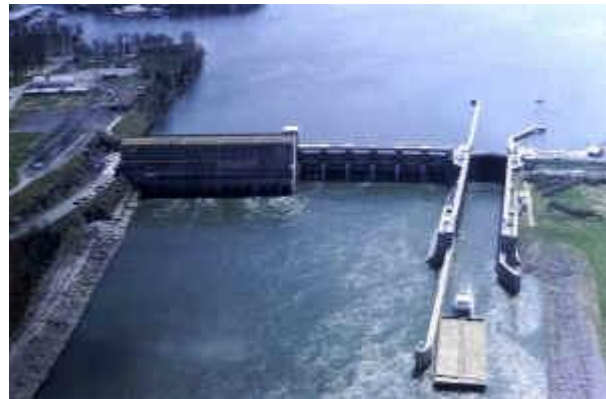
Figure 4-4a. Old Hickory Dam
